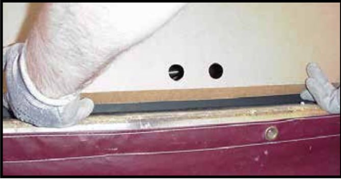
Figure 13.6 Folding Bottom Flap
