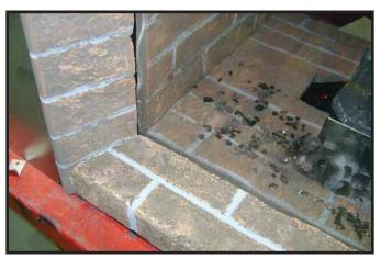
Figure 14.27 Outer Hearth Installation
