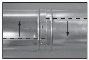
Figure 10.10 Rotate Seams for Disassembly
