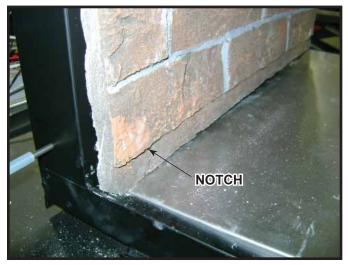
Figure 14.14 Notched End of Side Refractory
