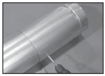
Figure 10.7 Screws into Slip Section
