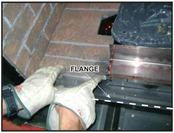
Figure 14.17 Positioning Left and Right Middle Base Refractory
