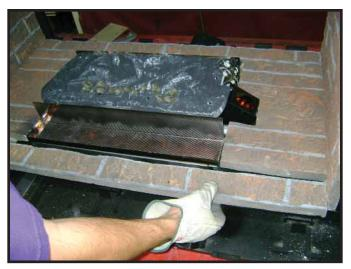
Figure 14.18 Positioning Outer Bottom Refractory.
