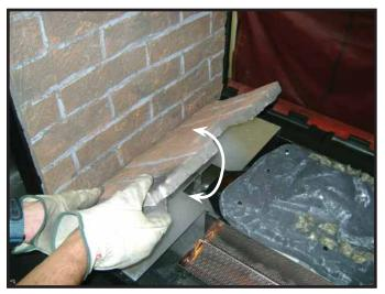
Figure 14.16 Positioning Inner Bottom Refractory
