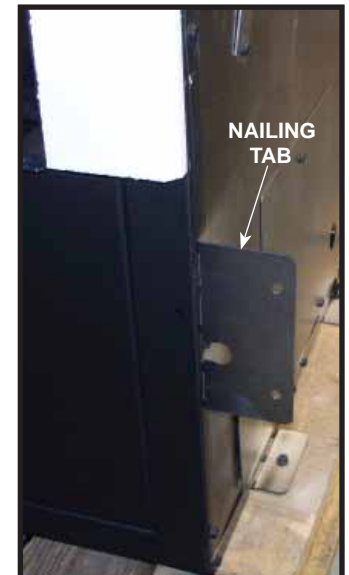
Figure 9.4 Nailing Tabs Installation Position
