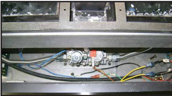
Figure 11.1. Valve Pressure Taps.
